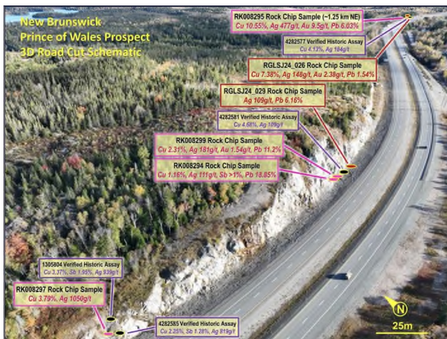
Figure 2 – Prince of Wales roadside cutting with exposed mineralization (Source of Map: Riversgold press release on ASX dated January 29, 2025)
